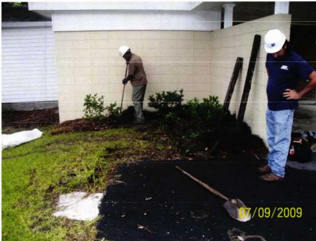
Picture 1: Location of UST 1373Dove prior to removal.
